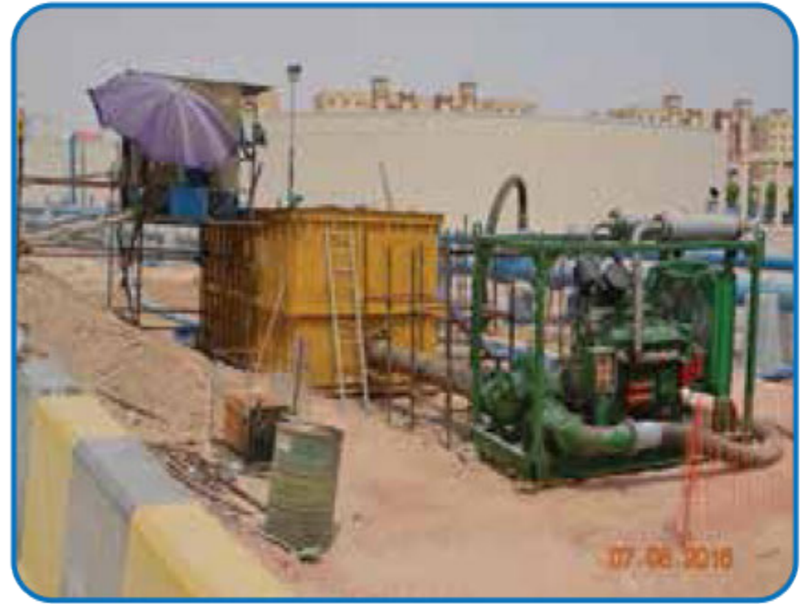
Flushing by open loop system
