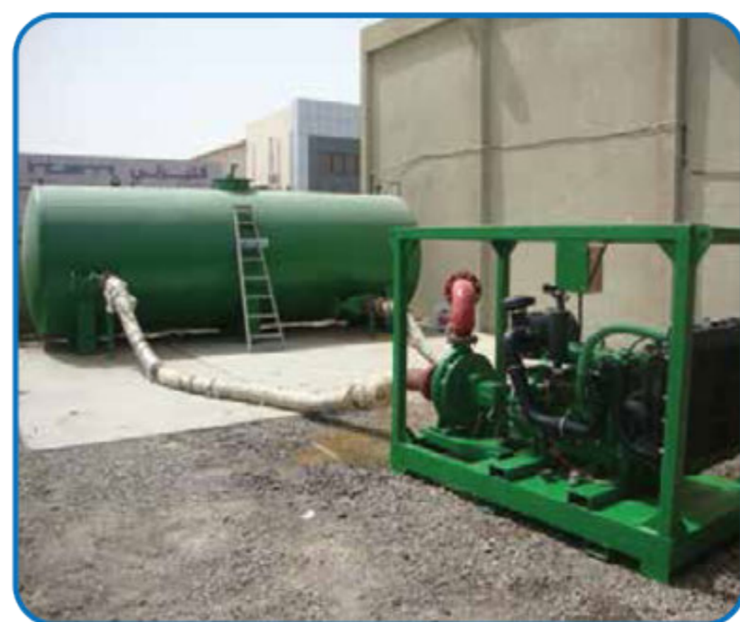
Diesel driven centrifugal pump on test
