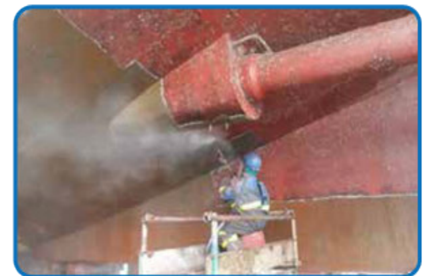
Hydro-blasting of underwater area
