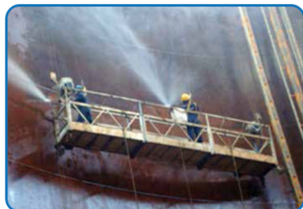
High pressure internal cleaning of tanks
