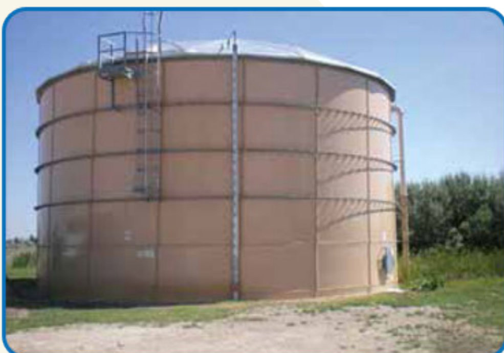
Hydro testing of storage tanks
