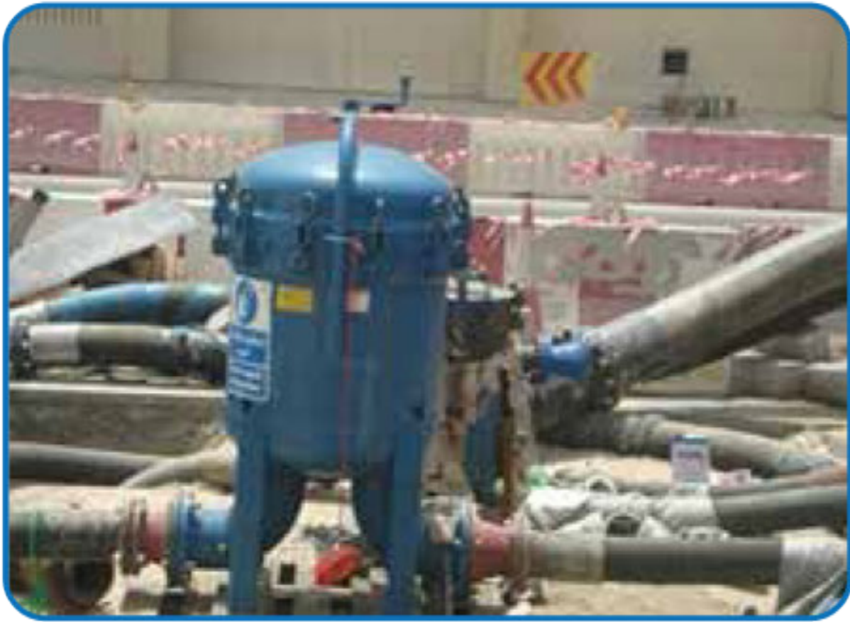
Typical multi-bag filter skid
