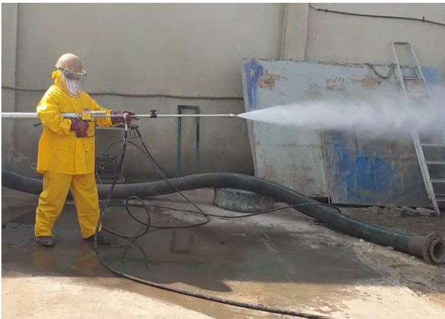
Water jet cleaning of heat exchanger tubes
