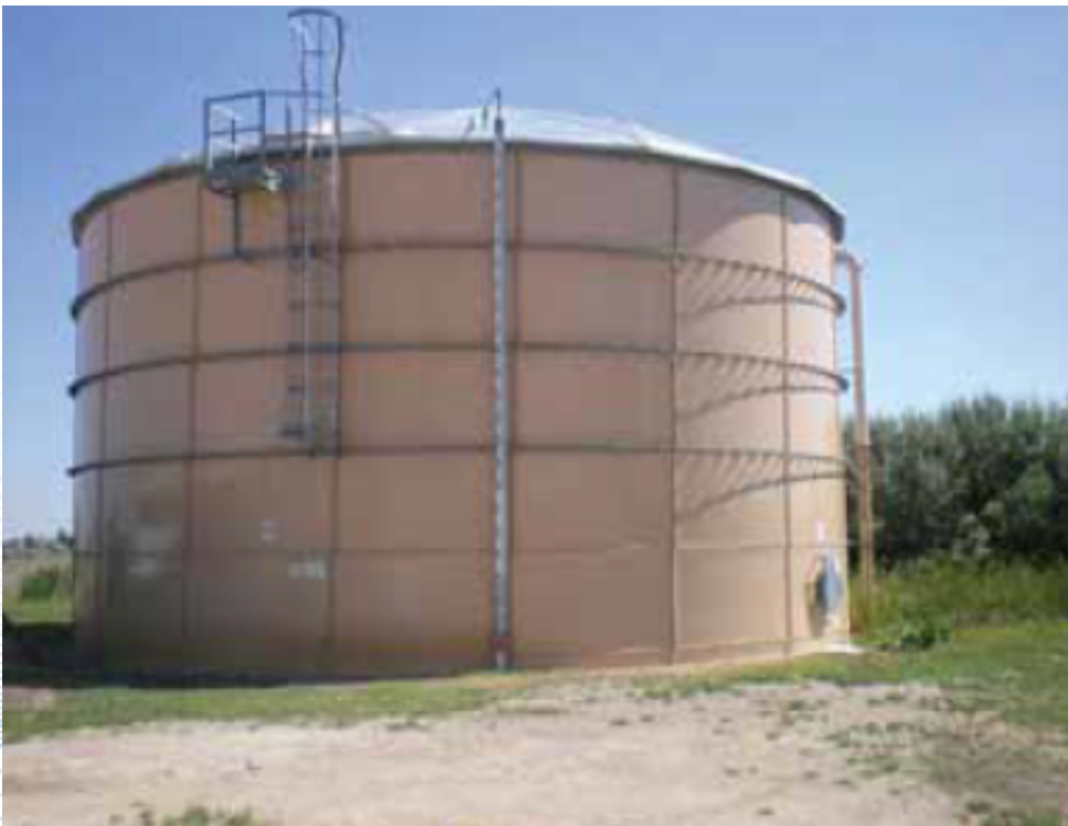
Hydro testina of storage tanks
